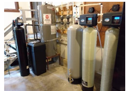
ECOsmarte System pictured with Salt Softener on Indoor Hot Water with 400ppm CALCIUM.
