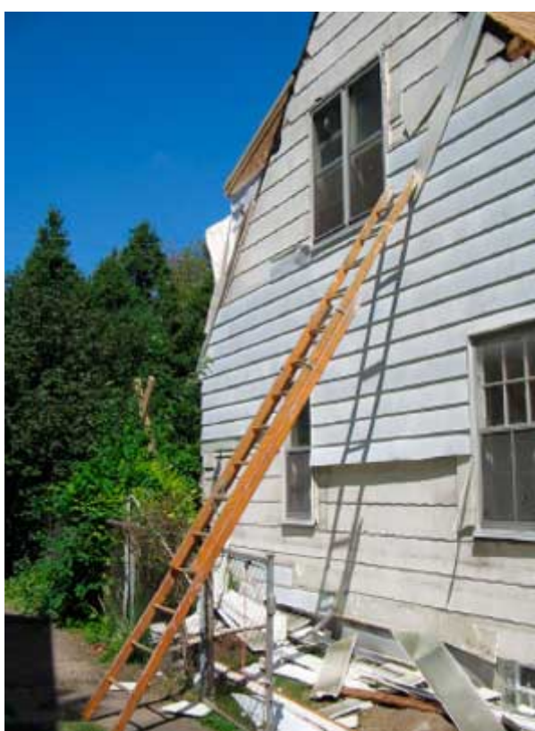
Figure 1. Siding being removed, ladder propped against fence.
