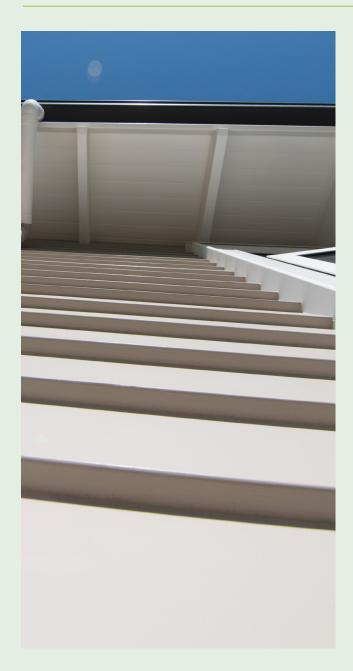
Timber weatherboards should be cleaned on a regular basis and at least once a year. Houses situated in a sea spray zone should be checked and could require washing two to three times a year. Particular attention should be paid to soffits and overhangs. Allowing mould, fungi and marine salts to build up by not washing could have a detrimental effect on both the paint and the timber substrate.
