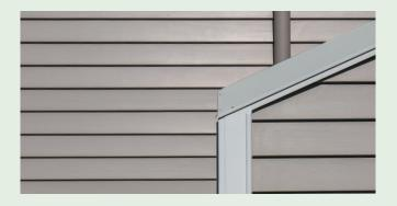
painted as soon as possible after installation, and no more than 90 days after installation. Primers cannot withstand extended periods exposed to the weather.
