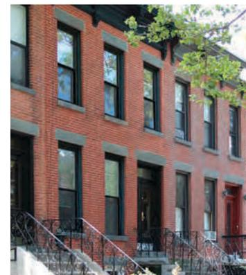
The front façade will be restored, with triple-pane simulated double-hung windows replacing the current vinyl-clad units. There are no Passive House-quality entrance doors that resemble the original, so the airtightness layer will wrap around the inner vestibule door, allowing a replica of the exterior door to grace the front.
