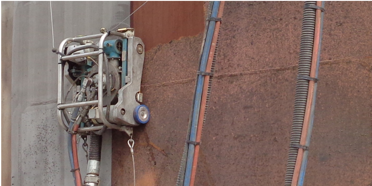
UHP robotic crawler operating on a storage tank exterior wall.
