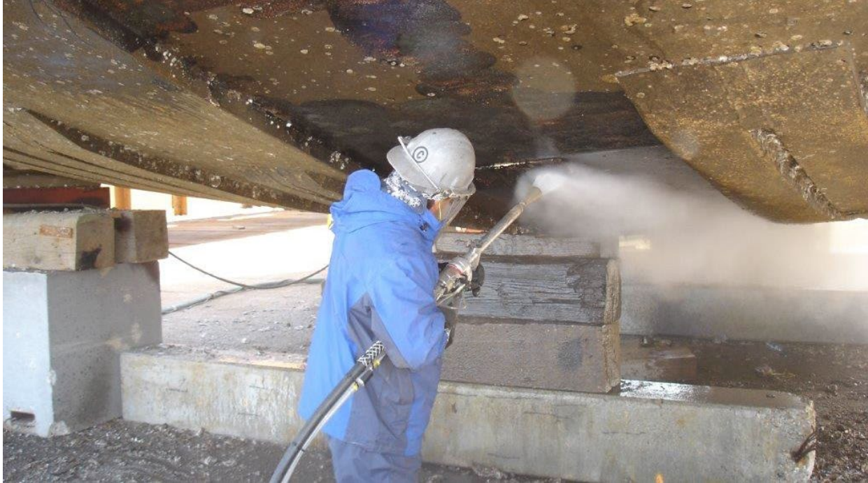
UHP hand lance waterjetting on a ship hull.
