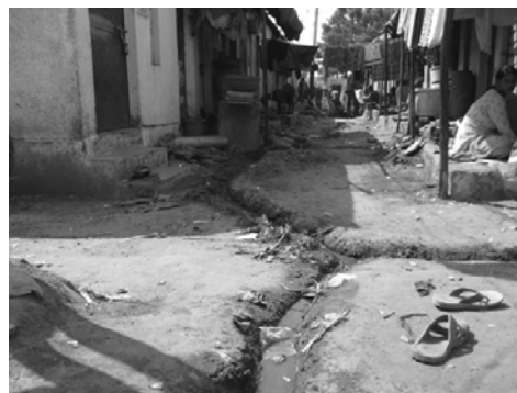
FIGURE 3: AD HOC GUTTERS ARE THE ONLY WAY TO DEAL WITH WASTE WATER IN IMDAD NAGAR, KHEDA DISTRICT
