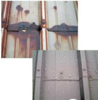
Figure 5 GE Enduris allows repair of panels with superficial rust
