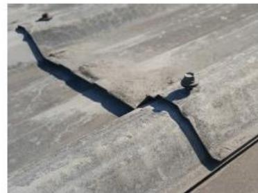
Figure 3 Corroding and Loose fasteners
