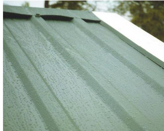
Figure 4 Silicone coated metal roof
