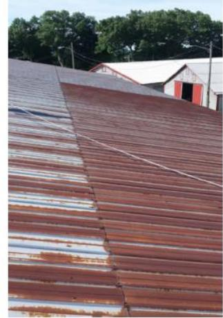
Figure 2 Corrosion can be either be Localized or Uniform
