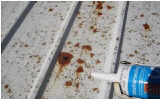
Figure 7 Fill small holes with sealant
