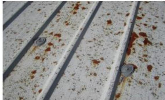
Figure 8 Cover fastener heads as needed
