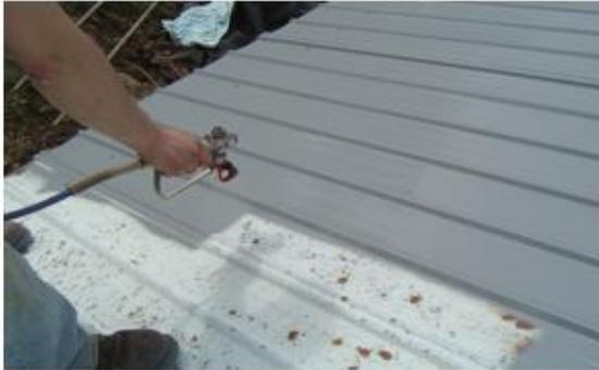
*Figure 11 Panels being coated*
