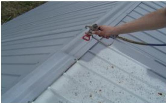
*Figure 13 Coating of ridge cap*
