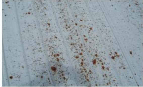
Figure 6 Metal roof before coating
