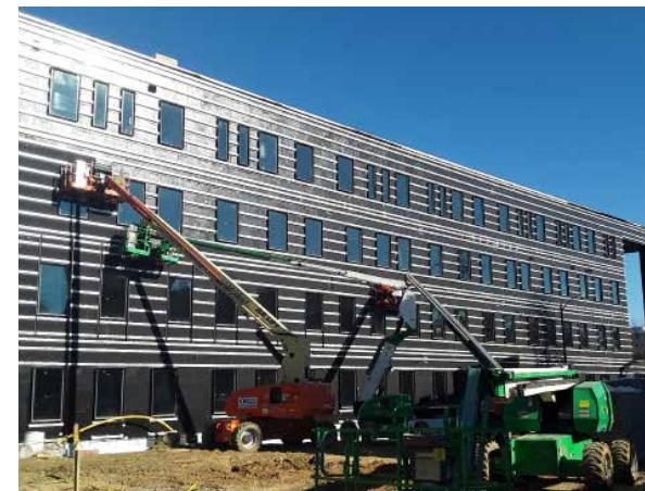
Work began in the spring, but soon, the Coronavirus crisis caused significant and immediate disruption. With the surfaces only partially coated, work was paused for several months. With an acrylic AWB coating, this delay would have likely posed a significant problem, as the product typically needs to be applied to surfaces within a strict time period, or otherwise require recoating.
