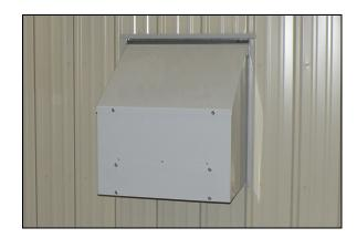
The Diversified Control **Free Air Cooler** is designed to save energy while maintaining a well regulated environment inside of a shelter. This is done by monitoring the inside and outside environments and intelligently choosing the least expensive mode of operation while limiting the inside environment to a user set temperature range.
