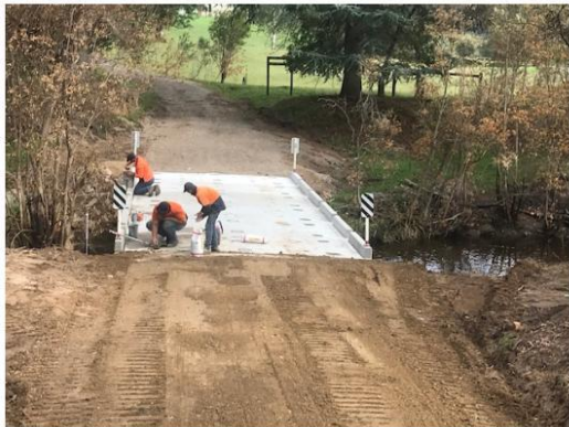
Repairs to the bushfire-damaged bridge at Reeds Road, Goongerah, were completed. The timber deck was replaced with precast concrete panels, spanning 13 metres x 4.2m.
