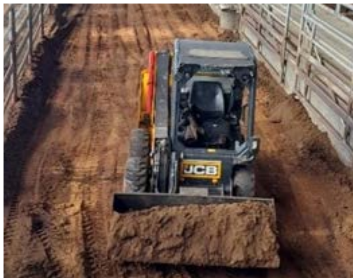
Ripping up and remove the old soft floor material ready to be replaced.
