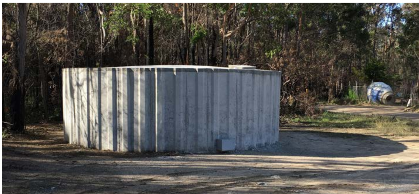
46,000L concrete static water tank in Mallacoota
