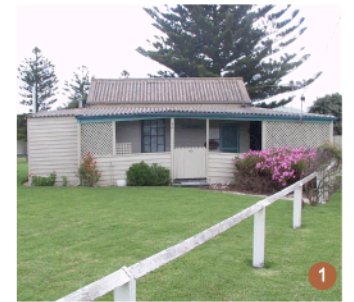
Typical older cottage
