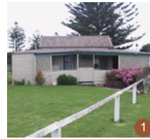
Typical older cottage
