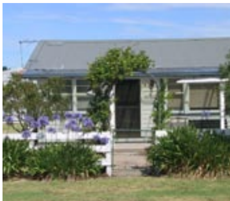
Cottage in older part of Seaspray
