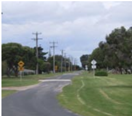
Intrusive powerlines and traffic calming
