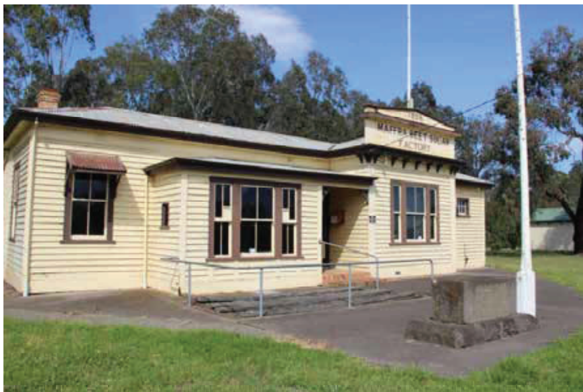
Figure D1. The facade of the former office, comprising the parapet to the projecting bay, and entrance in the section to the left. In front of the office is the original weighbridge, a foundation stone for the Beet Sugar Factory and early flagpole.
