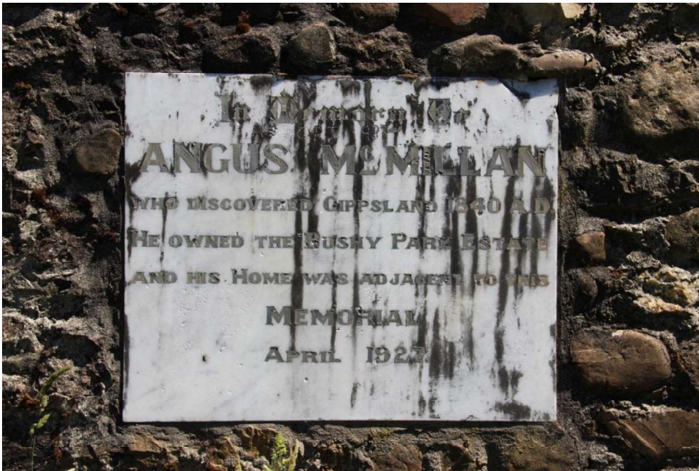
Figure D2. Detail view of the white marble plaque with incised lead lettering, and black staining.
