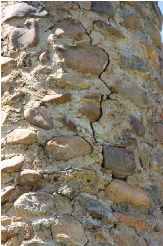
Figure D4. Detail showing the cracking to the tapering column, travelling around the small stones allowing water in.
