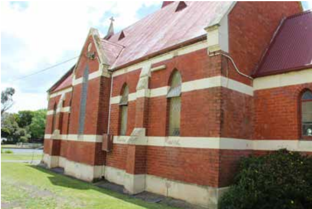
Figure D3. The south elevation. The side elevations of the nave are divided into five bays by buttresses with rendered coping. The central bay of each elevation has a (slightly projecting) gabled bay with a very tall pointed-arch window with leadlight. On both elevations, bands of decorative render (overpainted) run across the walls at sill level and impost level, (near the tops of the windows).
