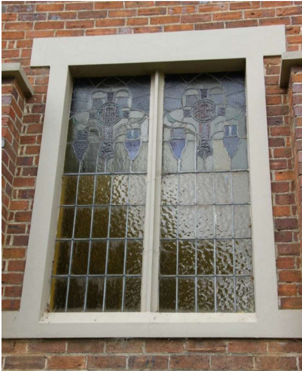
Figure D5. A detail of the windows on the south elevation (at the chancel end) show the geometric leadlight pattern to the bottom portion, and curvilinear detail of the Art Nouveau-inspired leadlight to the top.
