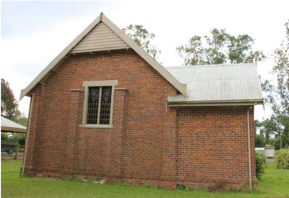
Figure D4. The rear (south) elevation has a jettied section at the top of the gabled end, clad with timber shingles, similar to the facade. Below is a double window of leadlight, flanked by a pair of buttresses.
