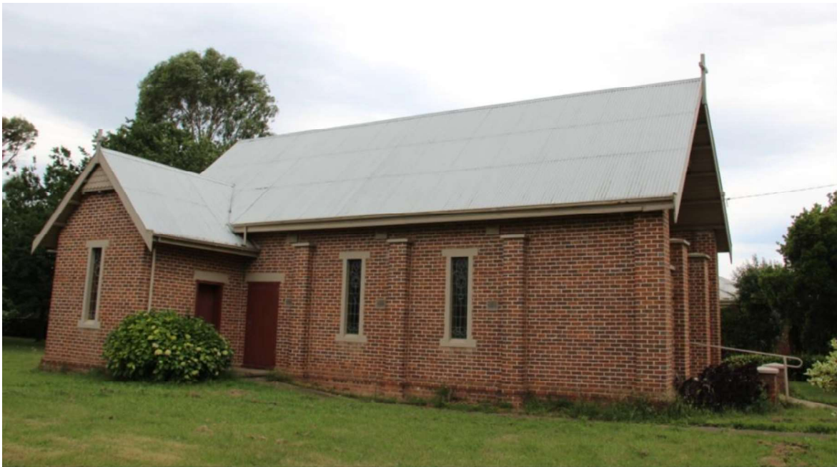
Figure D2. The east elevation. The side elevations comprise five bays, broken up by narrow engaged pilasters with a rendered cap. A vestry with a gabled roof projects to the east from the rear of the church, with the same treatment as the nave.
