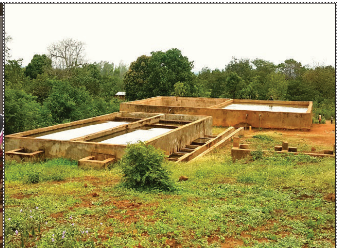
Mbadzi Water Treatment Works (2017)
