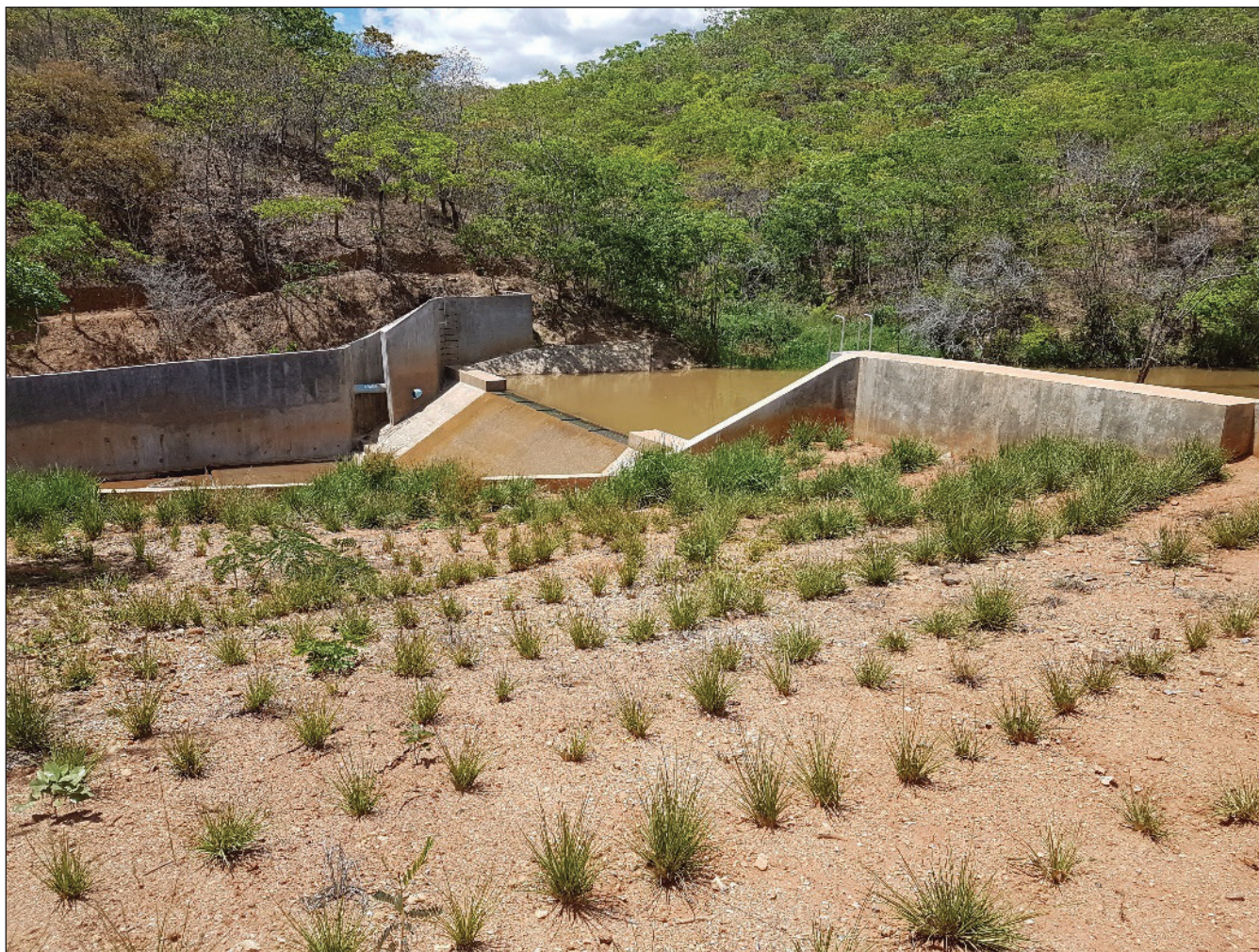
Photo 5.1 Kalenge Intake Weir
