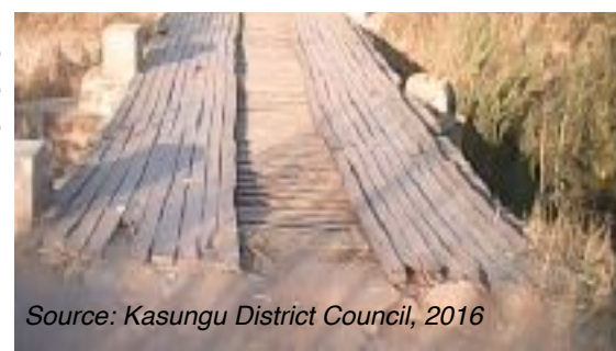
Photo 12: Timber-decked bridge
