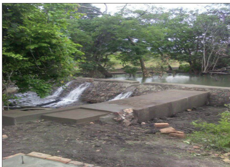
Figure 4.11 Weir for Liweredzi Irrigation Scheme
