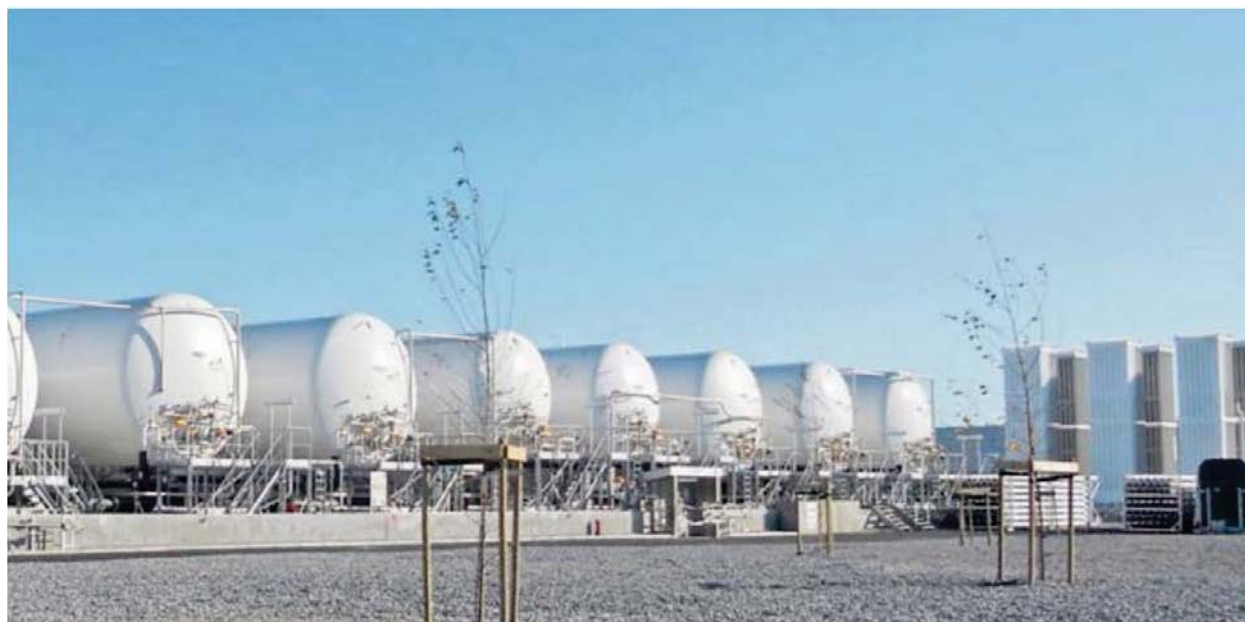
Figure 9 – LNG Terminal with Pressurized Tanks
