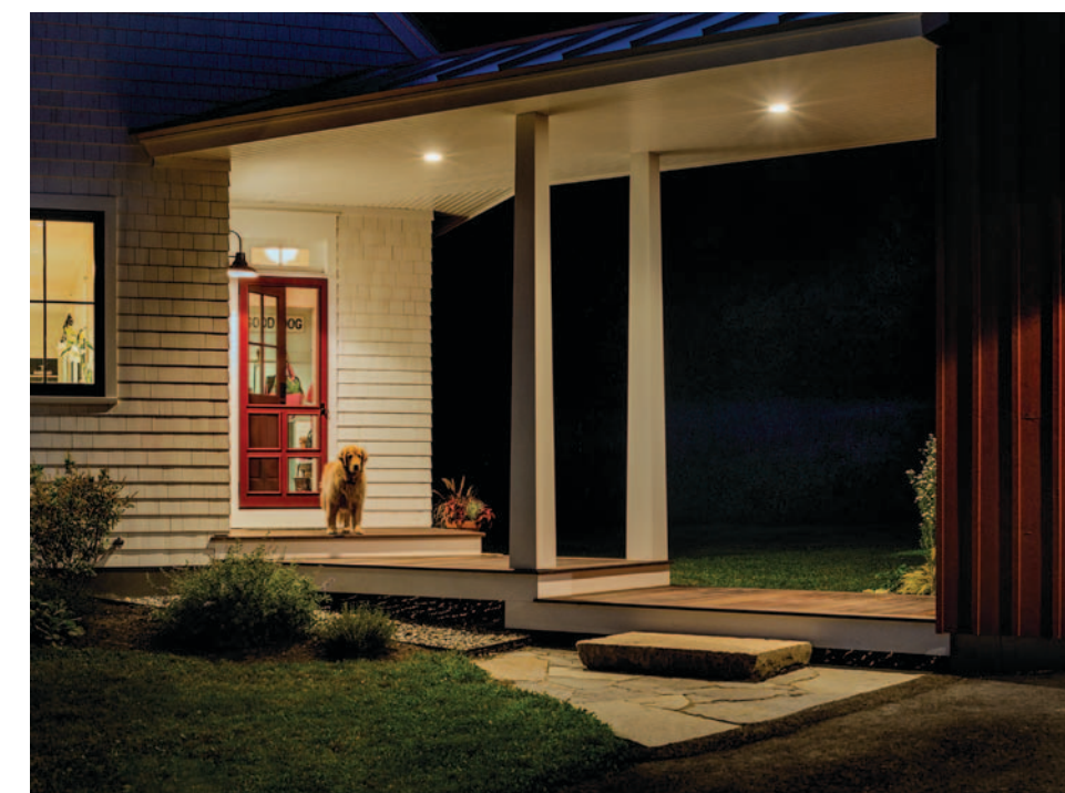
Covered connection. A sheltered walkway links the house's back entrance with the garage, about 20 ft. away. LVLs held up by tapered columns support the roof.
