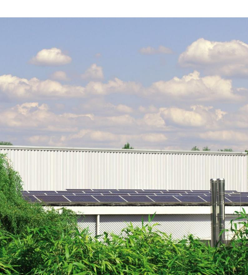
» The solar power system mounted on the roofs of our production **facility features a module area** of more than **1,940** m², **producing a nominal capacity of 273.36 kWp.** It has been generating electricity for more than three years now.
