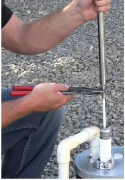
Reinstall the pump head and riser tube. Secure it firmly on the stainless nipple that is attached to the topmost drop pipe.
