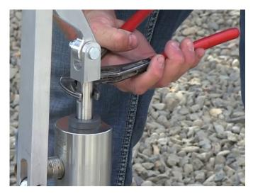
Using the 3/16" Allen wrench, loosen the pinch bolt and the 3 mounting bolts on the split flange enough to pull the pump head (including riser tube) up out of the well.
