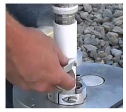
Lower the riser tube so that at least 6 inches of riser tube are below the split flange on the cap. Tighten the pinch bolt and 3 mounting bolts (right).
