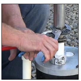
Lift the riser tube (and pump head), And then remove the safety tool.
