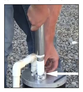
Use a channel lock to remove the riser tube and pump head. This allows access to the 3/4" stainless rod. **Do not** remove the stainless nipple (i.e. the short steel tube connecting the pump head to the top drop pipe).
