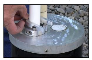
Then, slowly lower the bell end of the top drop pipe onto the safety tool (below).
