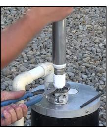
Disconnect the existing, 24", stainless steel rod from the topmost sucker rod. Install the 36" rod in its place.
