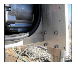
Screw the four mounting bolts (1/4-20x3/4" SS SHCS) through the holes just aligned, fastening the mounting plate to the pump head. (Left.)
