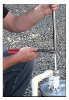
Reinstall the pump head and riser tube. Secure it firmly on the stainless nipple.
