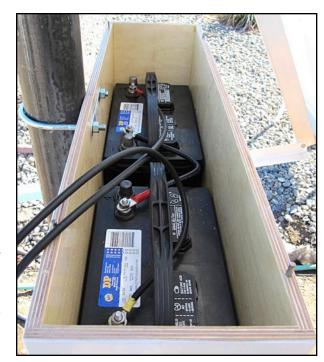
Notice that one of the ring terminals is larger in diameter than the other, 3/8" and 5/16". The 5/16" ring terminal attaches to the empty negative post of the first battery and the 3/8" ring terminal to the empty positive post of the second battery.
