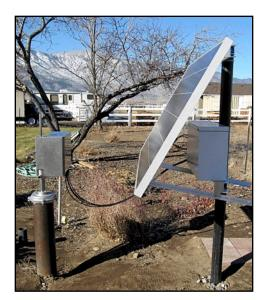
The batteries need to be kept clean and dry at all times, out of the rain, snow, ice, and direct sunlight, to increase longevity. The battery enclosure should be high enough off the ground to avoid rain runoff and snow accumulation.
